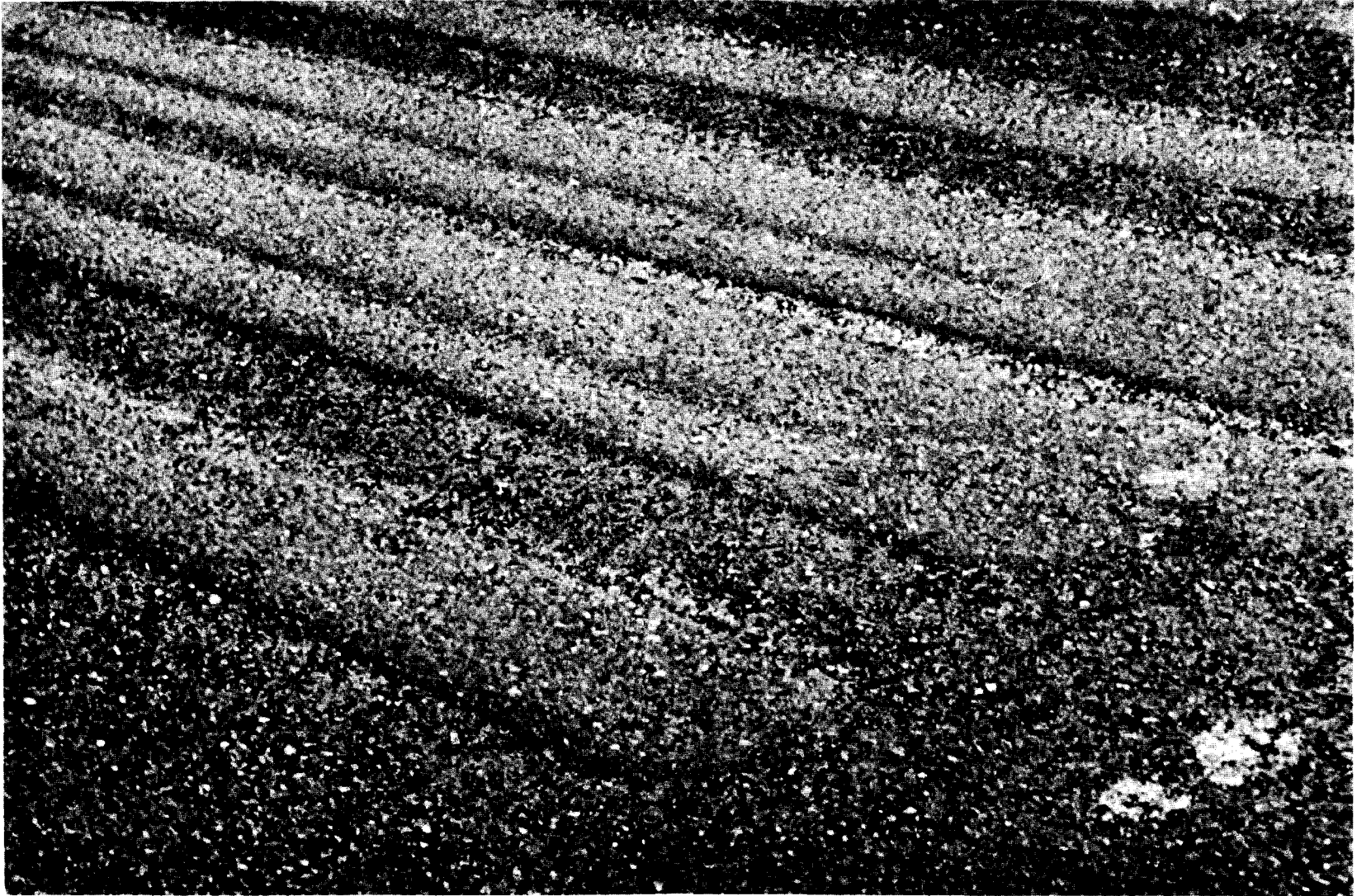
Figure 7—Illustrating tight surface texture provided by a pneumatic-tired roller.
